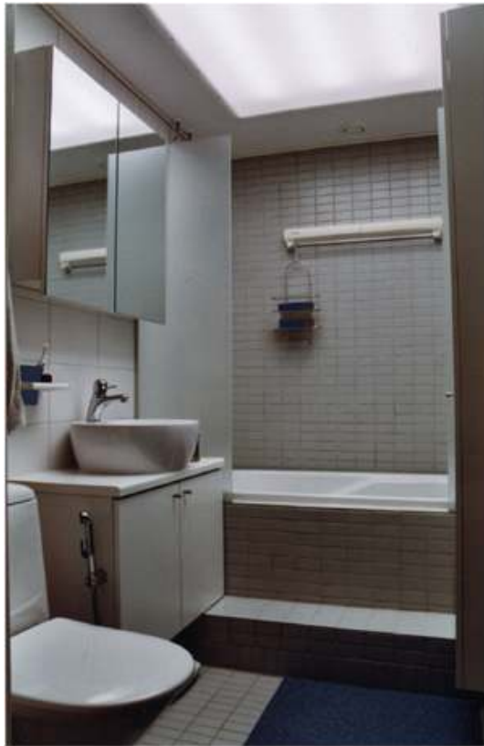
Lighted ceiling in bathroom
