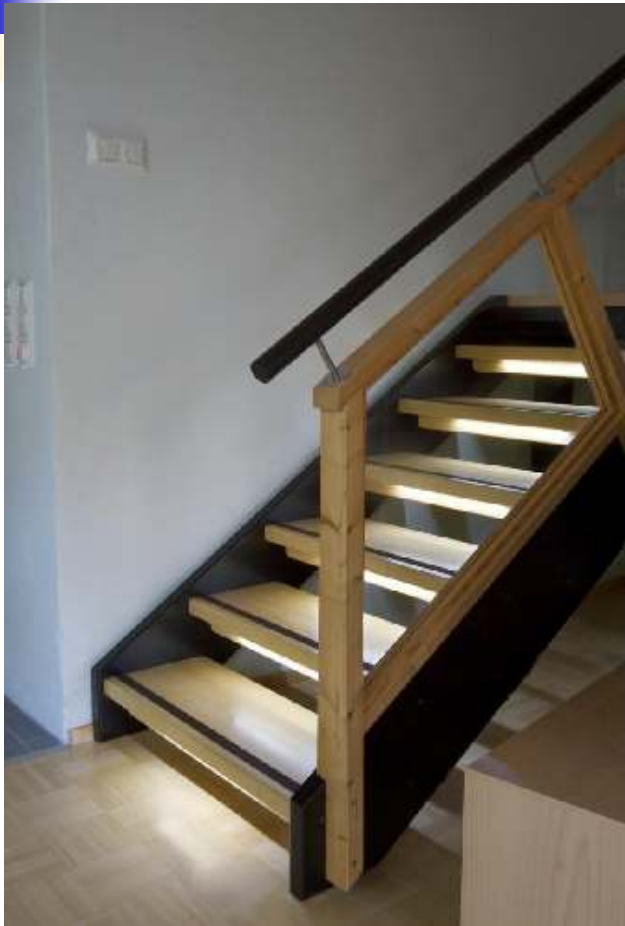
Stair lighting with LED
